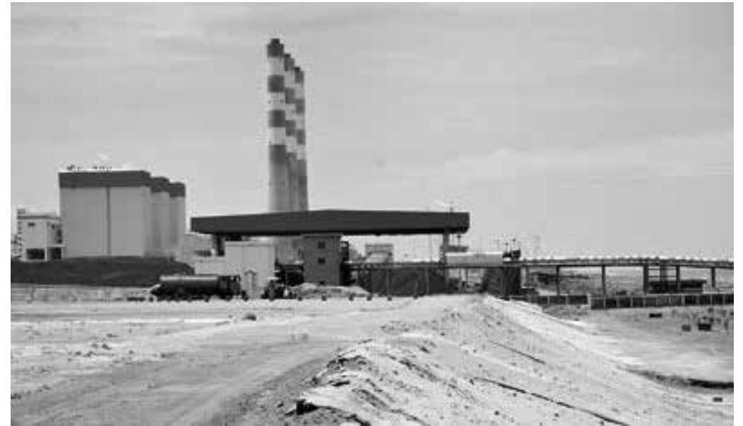
The crisis-ridden Lakvijaya coal power plant
